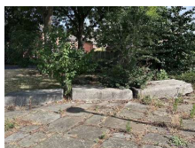
Existing granite stone blocks (to be re-arranged)
