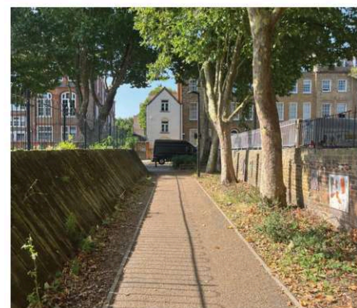
B Timber sleepers retaining wall
