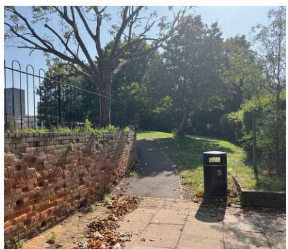
A Brick boundary, inaccessible route
